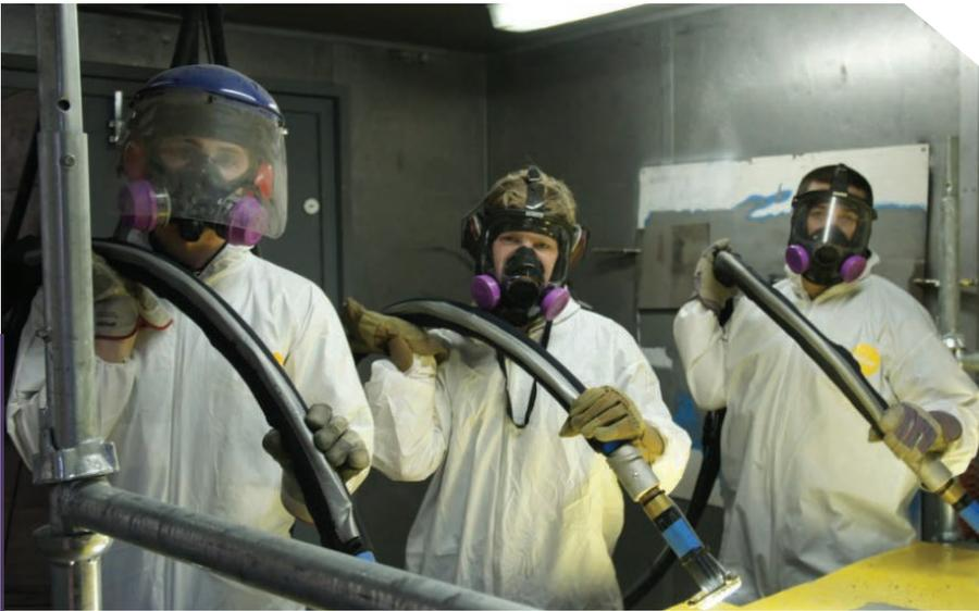
**LEFT: Low Dust Composite Abrasive Blasting in Ballast Tank**
