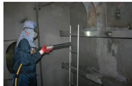
ABOVE: Low-dust abrasive blasting with recyclable encapsulated abrasive media (photo courtesy of Sponge-Jet, Inc.)
