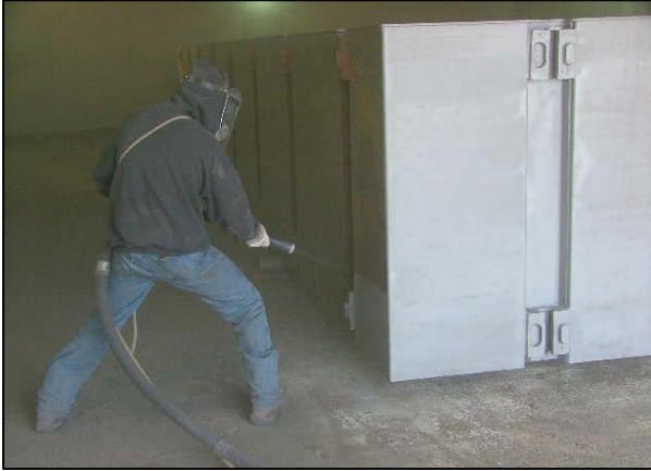
(Fig .5) Blasting sectional work barge with sponge-based composite abrasives
