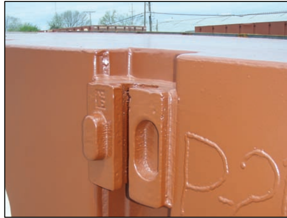
(Fig.7) After abrasive blasting and painting
