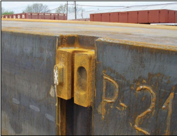
(Fig .6) Before abrasive blasting
