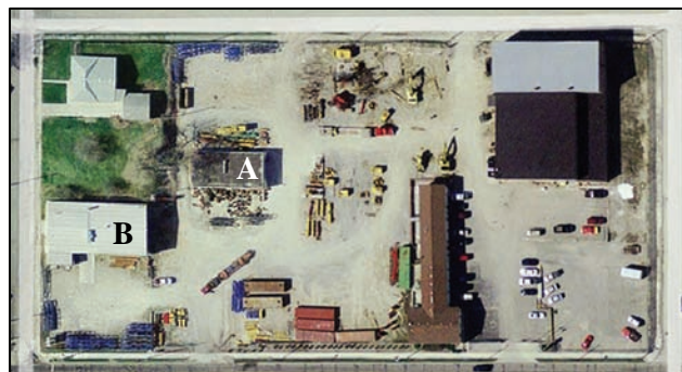
The barge manufacturer already had a blasting room (Fig. A) and painting room (Fig. B) to conduct spot repairs.
